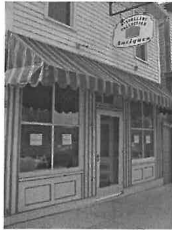
An example of a traditional fabric awning used on a historic building. Note the simple stripe, triangular shape and loose valance.
