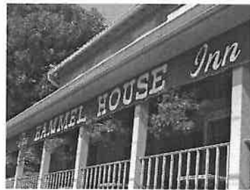
Awning sign at a porch
