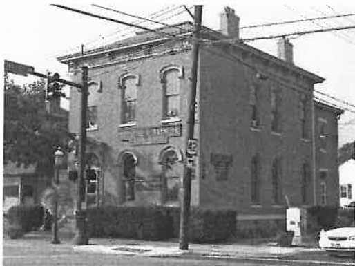
Several of the Landmark and Contributing Buildings are constructed of brick.
