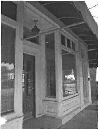
An original historic storefront in downtown Mason.
