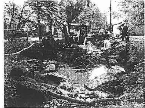
Urban stream restoration project under construction
