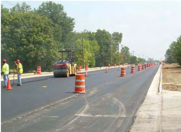
Western Row Road improvements will enhance a major east-west route in the city.
