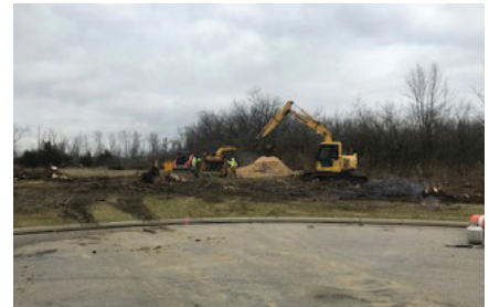
Moving Forward with Common Ground Ford Development Company clears land for future home of Common Ground Playground thanks to recent significant donations from TriHealth and the Scheeler Family.
